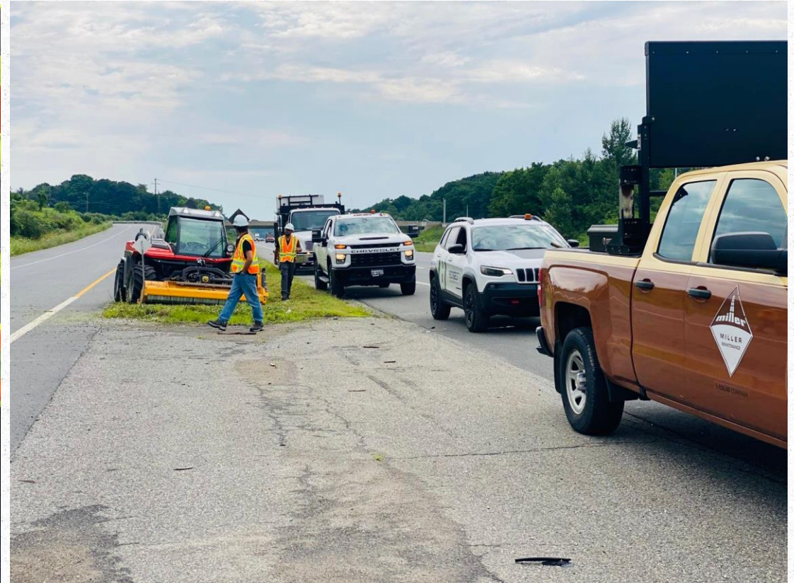
HWY 401 W Dixie Rd Interchanges
